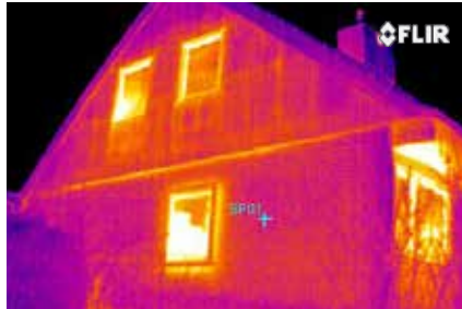
This thermal image shows an example of an insulation failure in a residential building that is used in Rockwool's thermography course.
