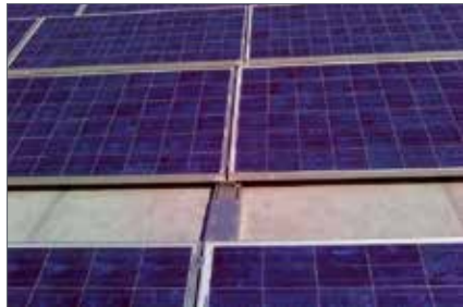
Visual image of a solar cell.
