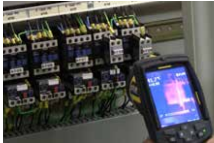
Inspection of a fuses in an electrical cabinet.
