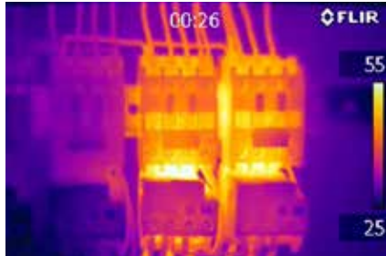
The thermal image clearly shows which fuses are too warm and will soon need to be replaced.
