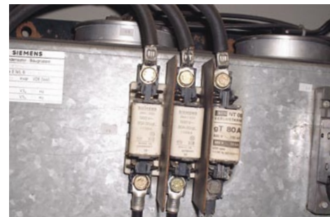
Fuse unit of a current compensation system
