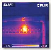
The thermal image clearly shows a defect or an overheated fuse. It can have very severe consequences. An entire production line can be shut down for several hours if this problem is not timely fixed.
