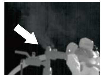
Captured SF 6 leak
